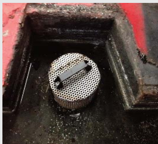
Special stainless steel sieve to cover round outlets in canal
