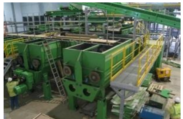
Residual Waste Treatment - AmeyCespa
