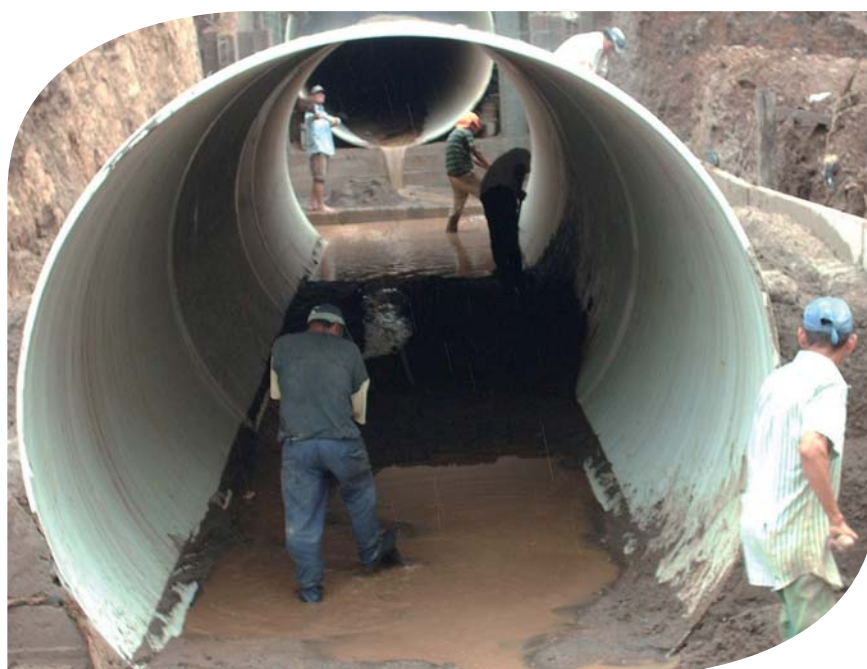
Salvador - Over 1,800 linear meters of Ribsteel piping with a diameter of 2,750 & 3,000 mm was installed in 2007 for the residential areas in Salvador
